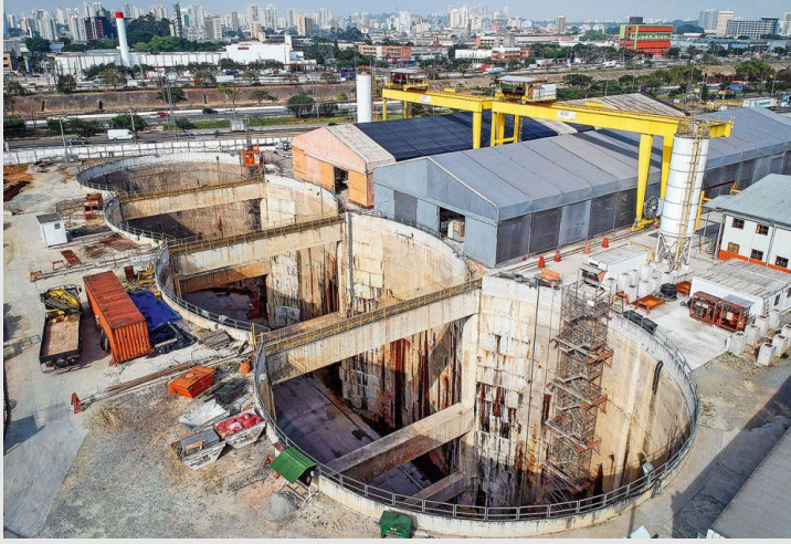
In the Picture, a construction site of Line 6-Orange
